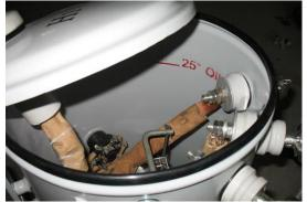
Care should be taken to re-seal the transformer so that moisture is permanently excluded from the interior. A pressure test using dry air or nitrogen, may conveniently be made through the pressure vacuum fitting, after removing Single-phase Distribution Transformer
