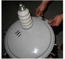
A recommended procedure for opening the transformer is to first bring the interior of the transformer to atmospheric pressure by venting the automatic relief valve pressure furnished allEVERPOWER on transformers. The cover band may then be removed. Natural rubber hose should not be used in the transfer of oil. The correct oil level at 25°C is marked on the inside of the tank.
